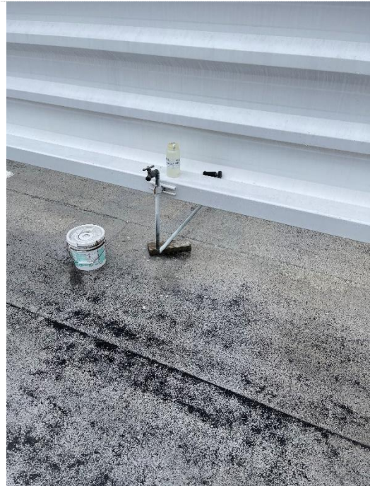
Photo #8: Rooftop hose bib
