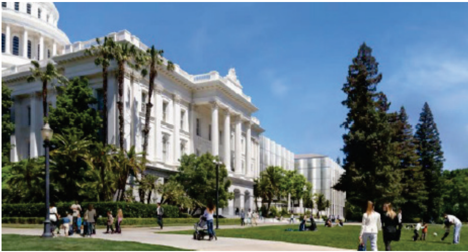
South Facade of Proposed New Glass Annex protrudes beyond the Historic 1874 Capitol.
