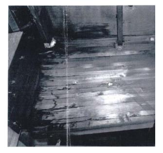
**Example of Language**: "Two glu-laminated beams have experienced crushing, etc. at one end due to years of water intrusion form the roof.... As a result of the end damage, the bolting of the glu-laminated beam to the steel bucket can no longer transfer the out-of-plane seismic loads.... This could lead to a partial roof and wall collapse during a seismic event. Consequently, the compromised glu-laminated beam ends constitute a current life safety hazard...."
