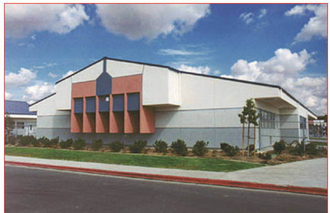
Typical Classroom Building
