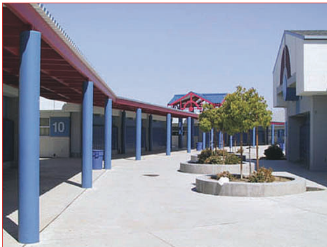
Pergola Style Walkways between Buildings
