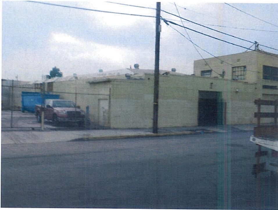
Southwest view of subject property.
