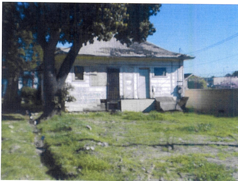
Easterly view of subject property from alley.
