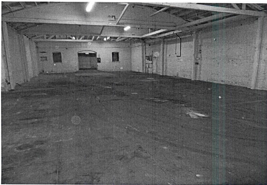
PHOTO NO. 7: Interior view of Interior view of shop area within building identified as 3828 South Main Street.
