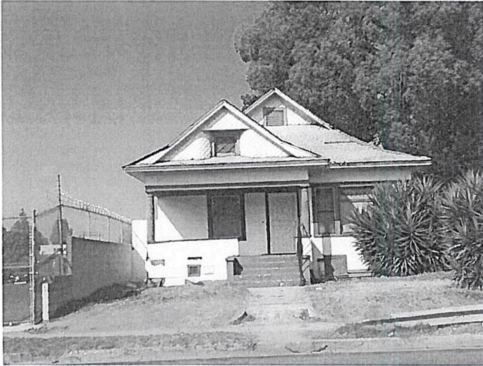
Westerly view of subject property from the front.
