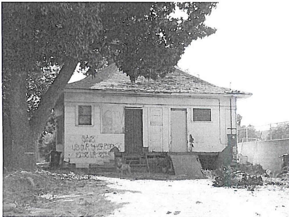
Easterly view of subject property from the rear alley.
