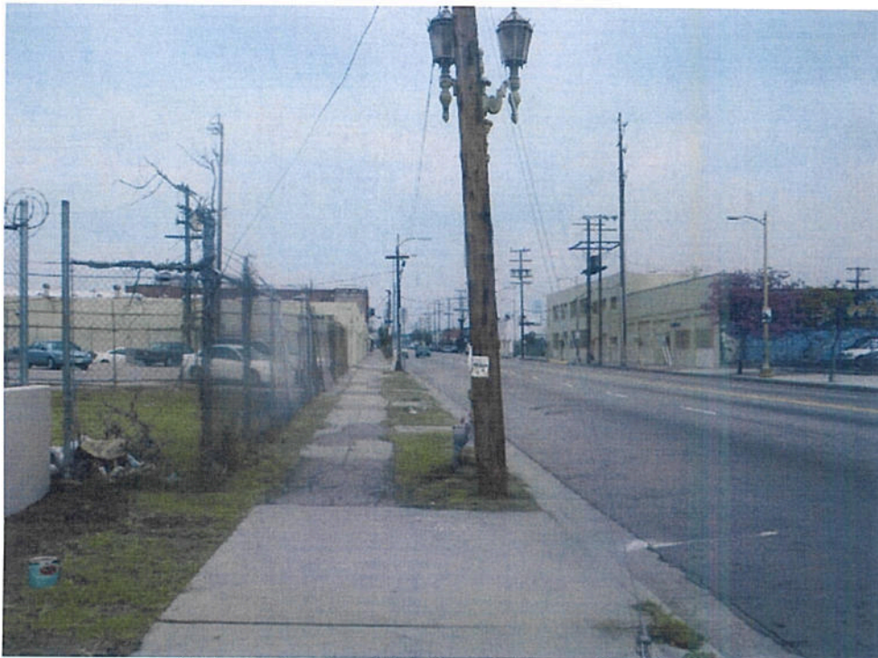
Northerly view along Main Street (subject parking at left).
