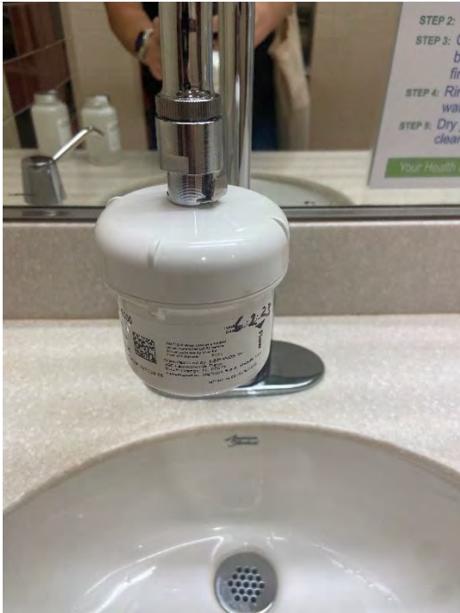
Photo #7: POU filter installed in restroom with new fixture
