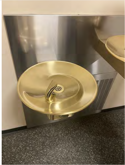
Photo #6: Newly replaced drinking fountain
