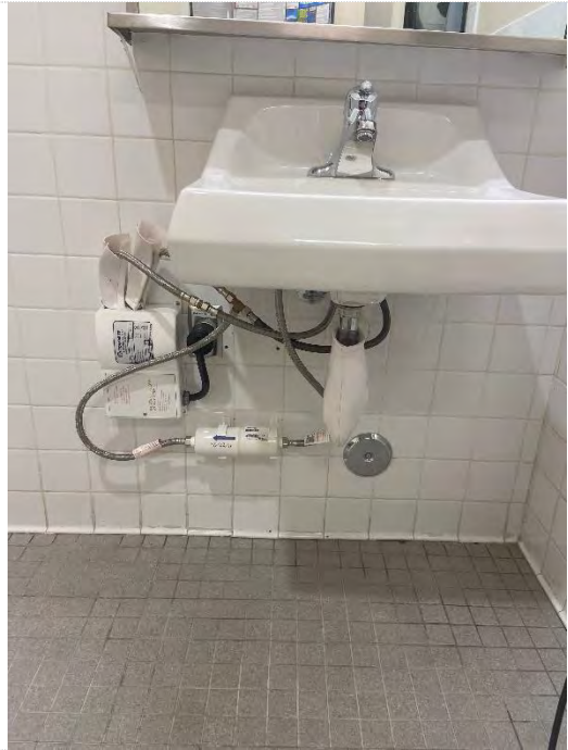
Photo #4: In-line filter and hot water heater – Suite 108 restroom sink
