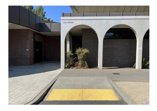
A curb ramp is the accessible link between the parking lot level and the walk that leads to the accessible entrance. Noncompliant curb ramps can be hazardous and a liability for the property owner. So, it is important to get it right.
