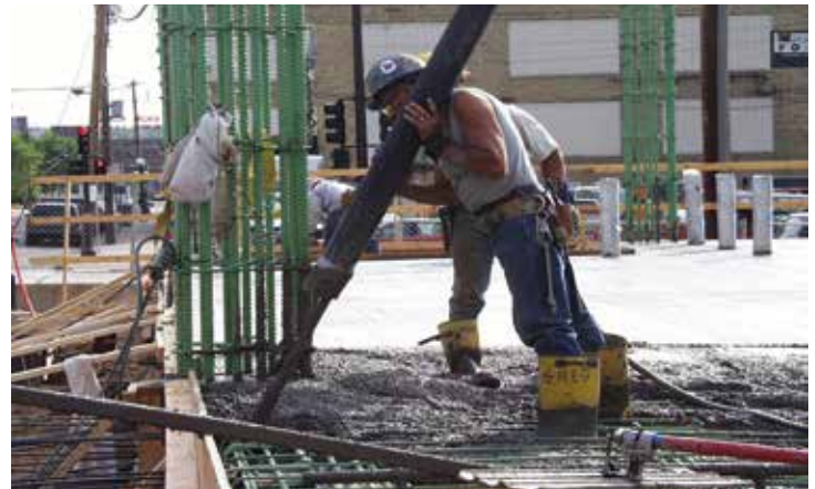
Placing Concrete
