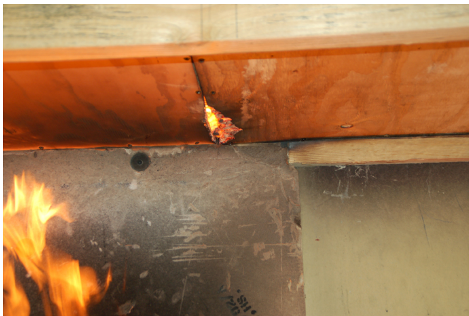
Figure 5. Flame penetration at a between-panel joint allowing for flame propagation to occur within the enclosed soffit cavity. This test was terminated prior to ignition of the soffit material and flame propagation to the fascia.
