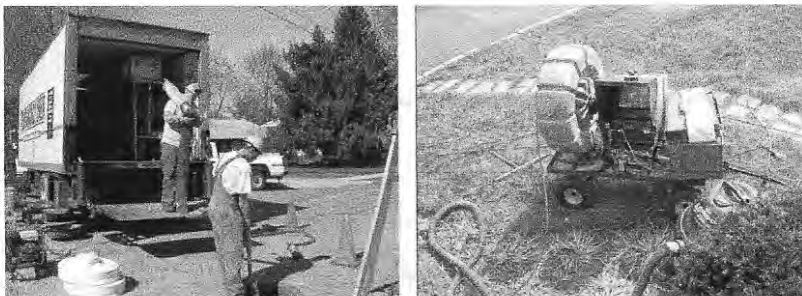
Figure A-25. Positioning of the Launcher. Left: Insertion through the Manhole. Right: Lateral CCTV Camera.
