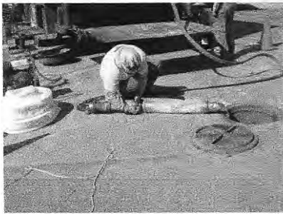
Figure A-24. Completing the Loading of the Launcher.
