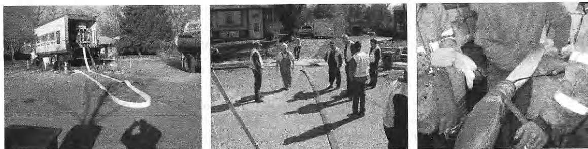
Figure A-23. Pulling the Liner/Bladder Assembly into the Launcher. Left: Both Tubes Laid Out on the Ground. Middle: Pulling the Cable Inside the Launcher. Right: The Assembly Entering the Launcher.
