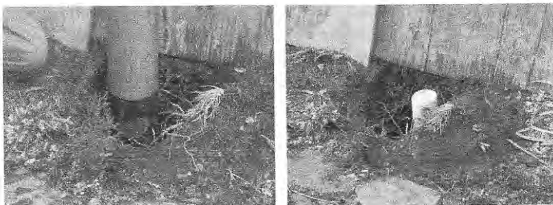
Figure A-17. New Cleanouts. Left: Pit Hydro Excavating. Right: Installed Vac-A-Tee® Cleanout.
