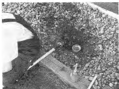
Figure A-19. Cleanout Ready for Pipe Cleaning.
