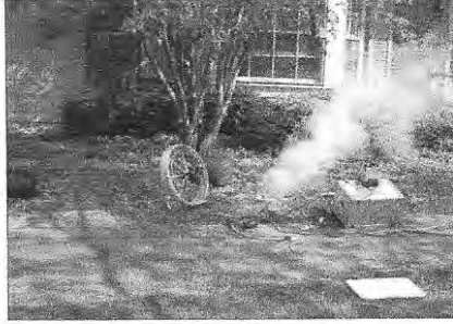
Figure A-27. Resin Cure. Left: Steam Hose Connected to the Bladder. Right: Steam Exiting at the Cleanout Near the House.
