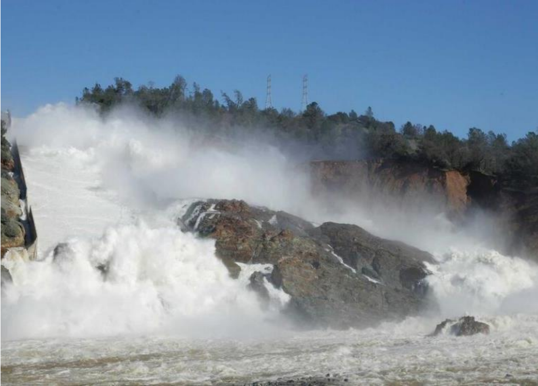
Water flows down Oroville Dam's main spillway on February 13, 2017.
