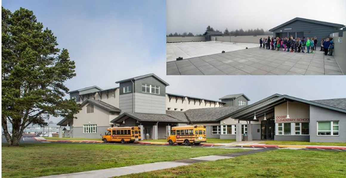
The first tsunami vertical structure in the United States: Ocosta Elementary School, Westport, Washington. The building is designed to withstand an earthquake and has a flat roof over the gym to accommodate up to 1,000 students and community members from a resulting tsunami.
