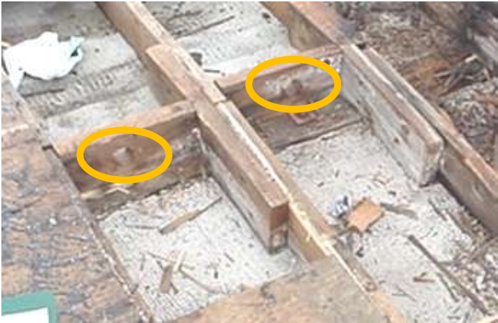
Figure 2-68: Enclosed Rafter Space Ventilation Holes at Ridge
