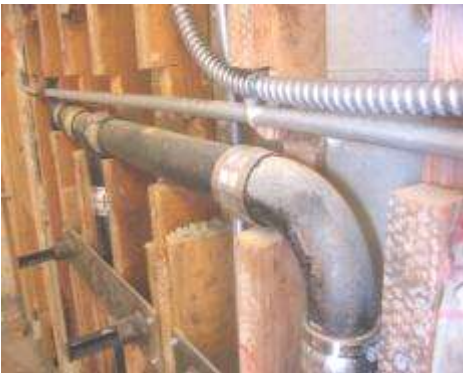
Figure 2-32: Unacceptable Notching
