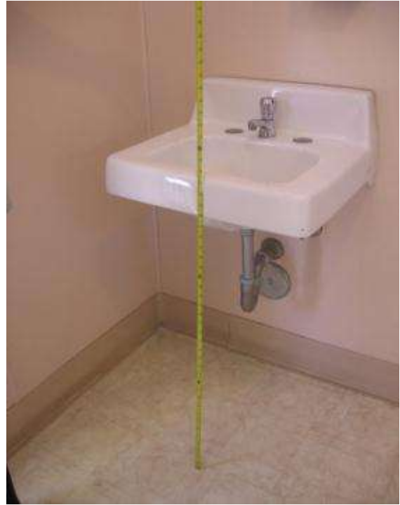
Figure 4-16: Example Measurement of Lavatory
