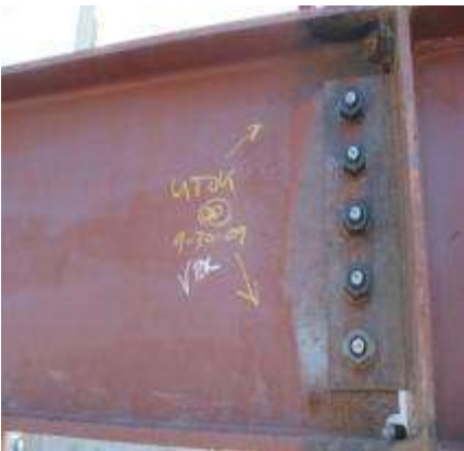
Figure 2-59: NDT Special Inspector Markings
