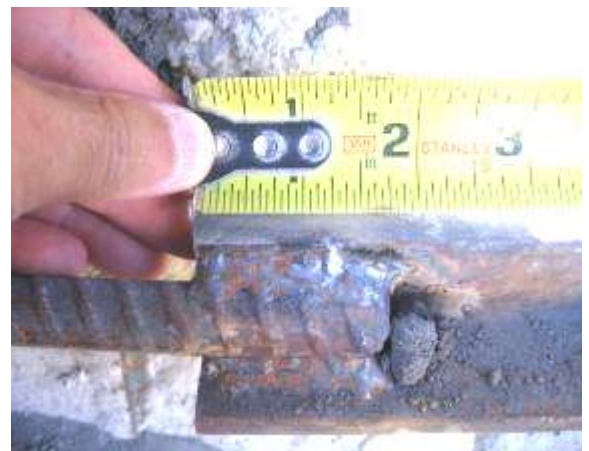
Figure 2-18: Verify Weld Lengths Per Requirements
