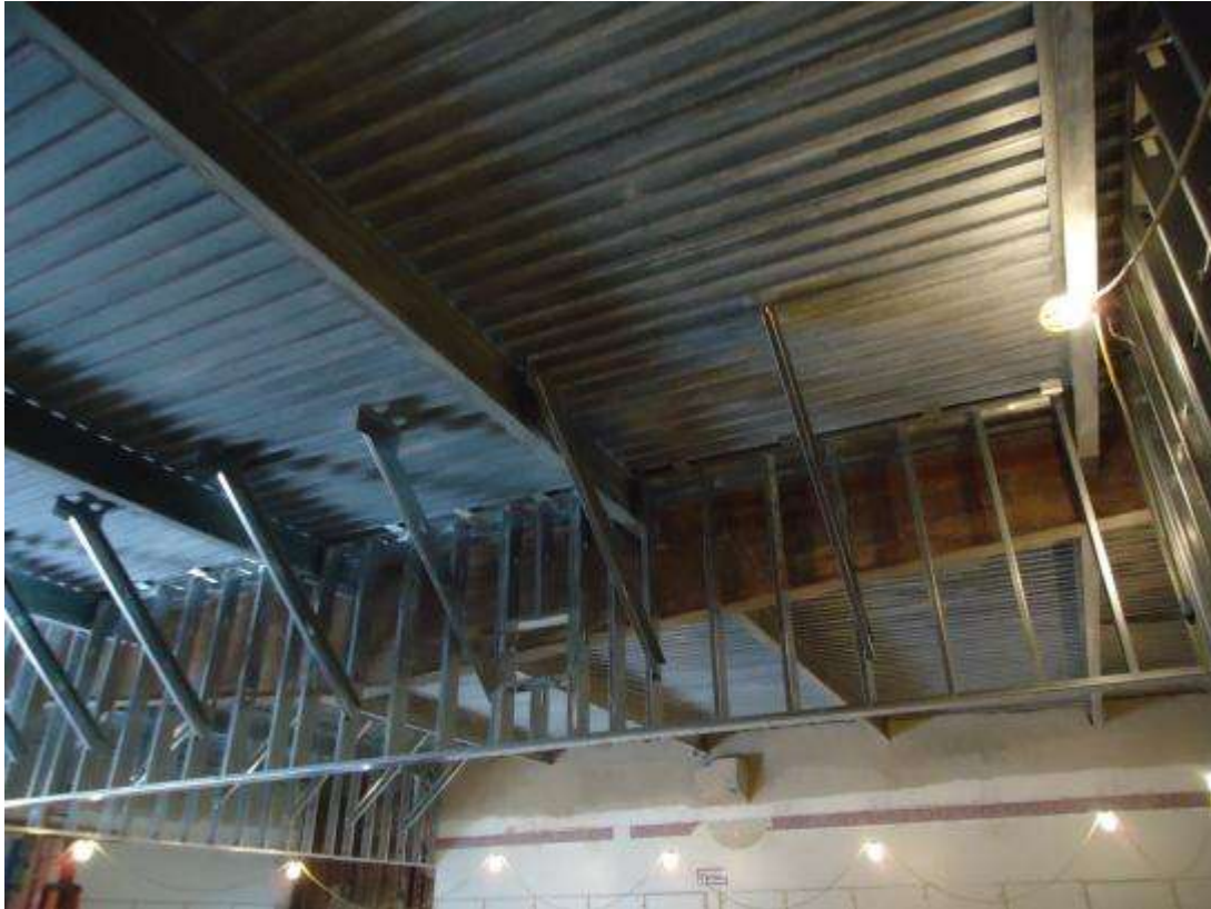
Figure 2-64: Example of Soffit Bracing
