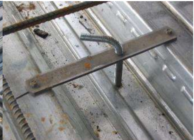
Figure 2-52: Concrete Deck Insert
