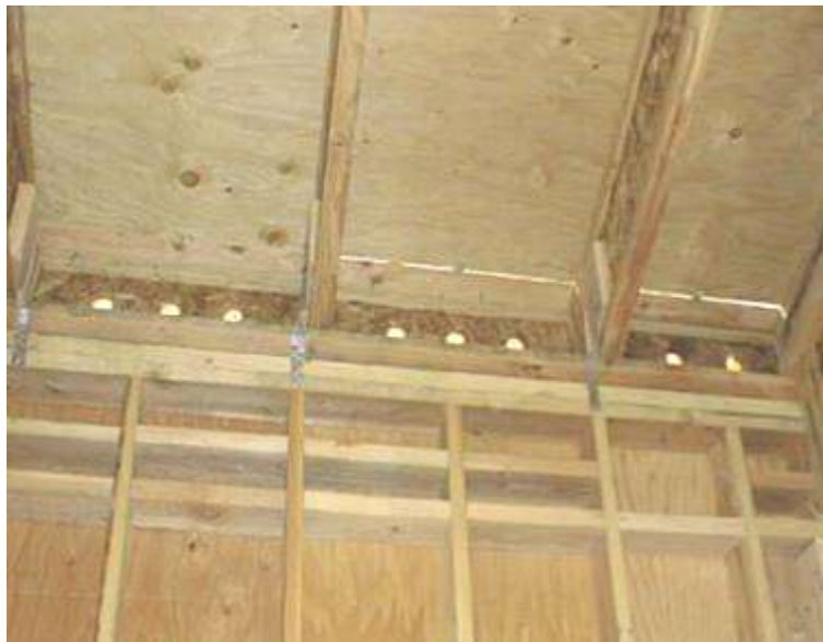
Figure 2-67: Attic Ventilation Holes
