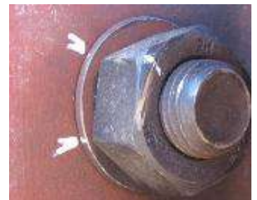
Figure 2-42: Improperly Match Marked/Torqued
