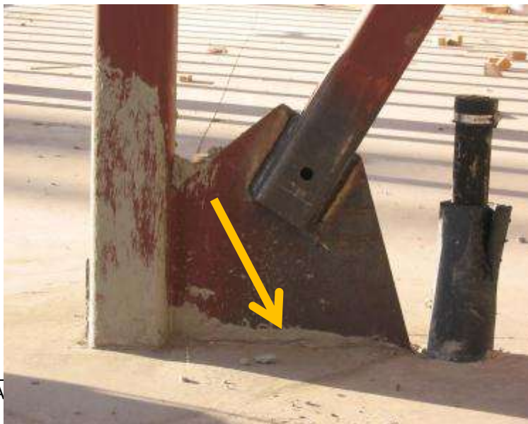
Figure 2-61: Concrete Slab at Gusset Plate
