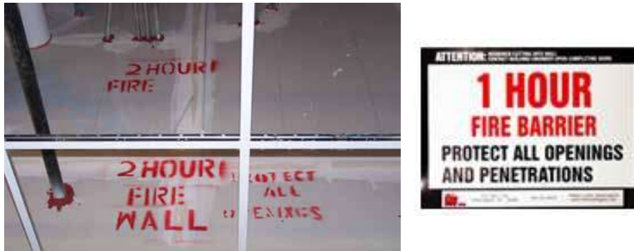
Figure 3-2: Examples of Fire/Smoke Rated Wall Identification
