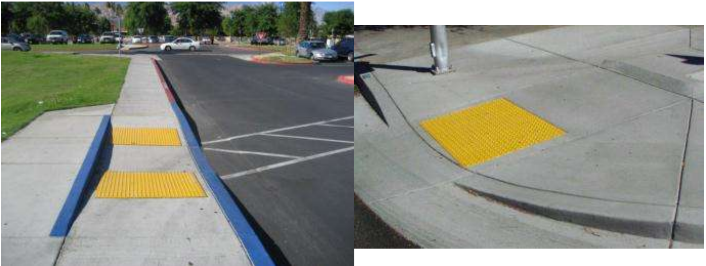
Figure 4-4: Curb Ramp Examples
