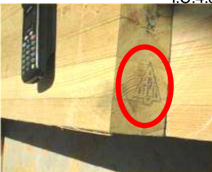
Figure 2-29: Glulam Special Inspection Stamp Example
