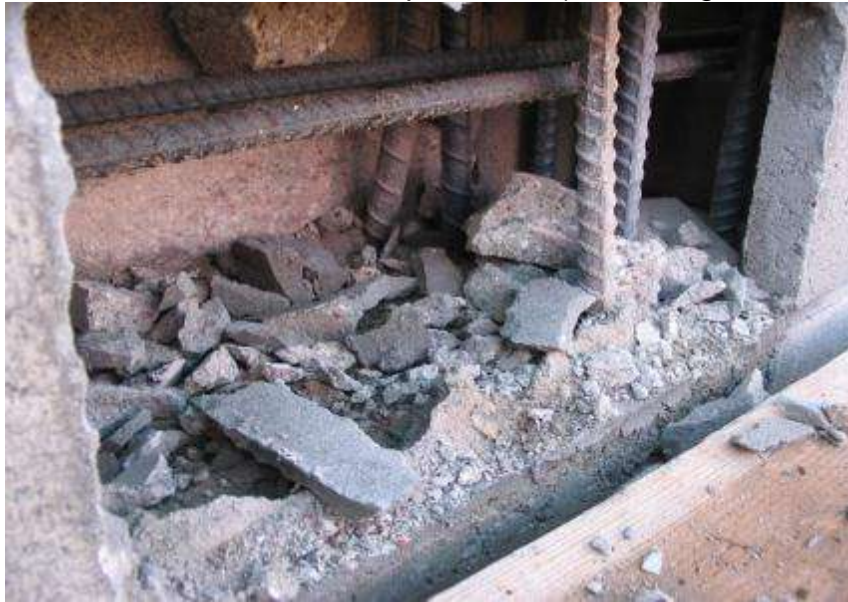
Figure 2-21: Cleanouts at Bottoms of Cells
