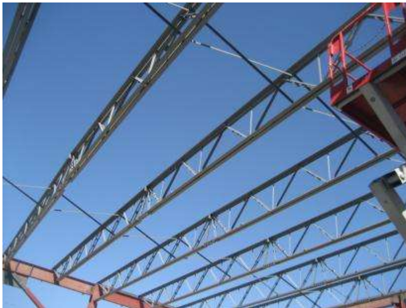
Figure 2-43: Steel Joist Bridging
