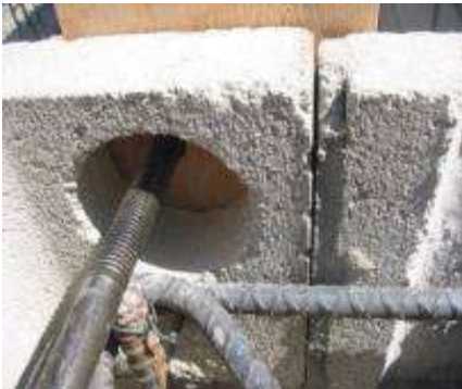
Figure 2-20: CMU Clearance at Bolt
