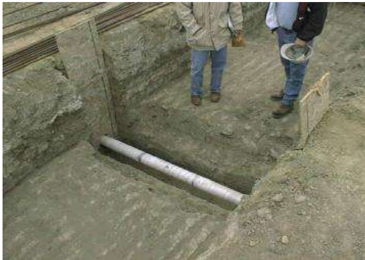
Figure 2-6: Pipe Through/Below Footing
