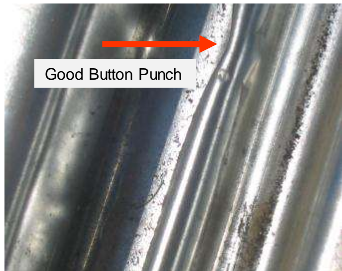
Figure 2-50: Good Deck Button Punch
