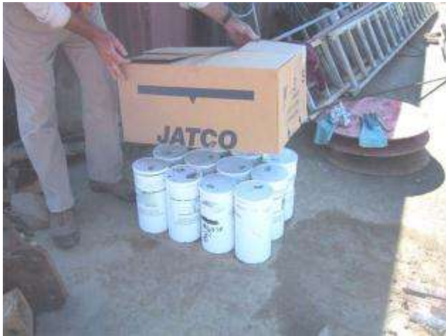
Figure 2-10: Improper Storage of Concrete Cylinders
