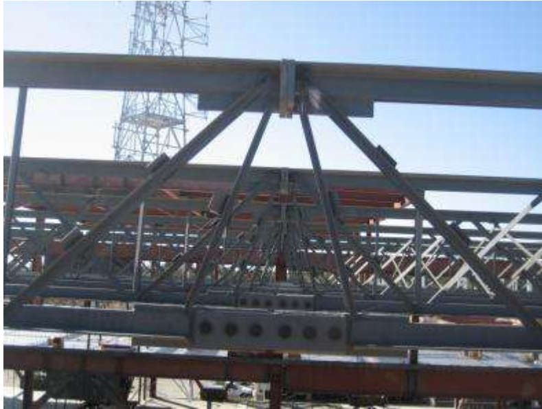
Figure 2-44: Field Splice of Steel Joists
