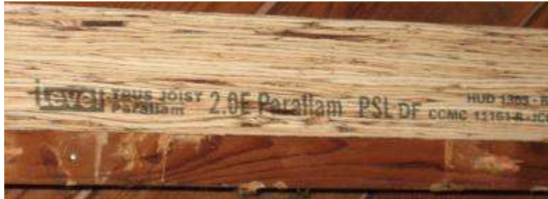
Figure 2-28: SCL Markings Example
