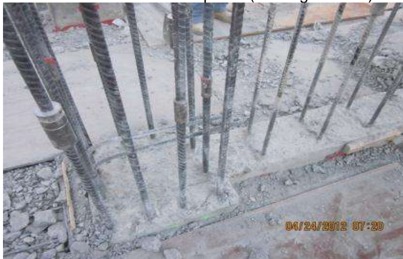
Figure 2-54: Steel Reinforcing Mechanical Splices
