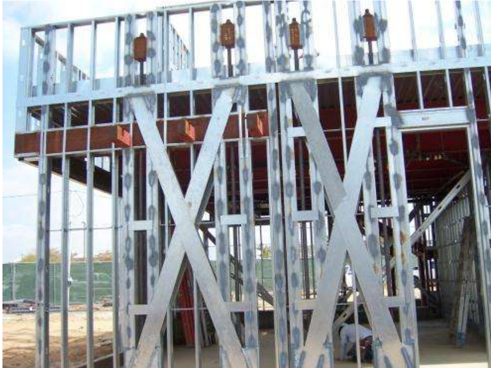
Figure 2-46: Example of Corrosion Protection at Welded Studs
