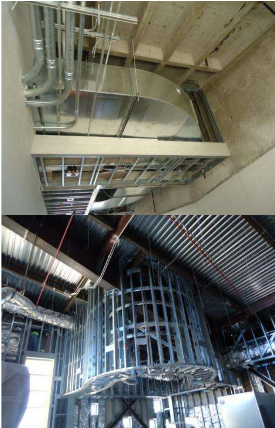
Figure 2-63: Soffit Framing at Ducts and Primary Framing
