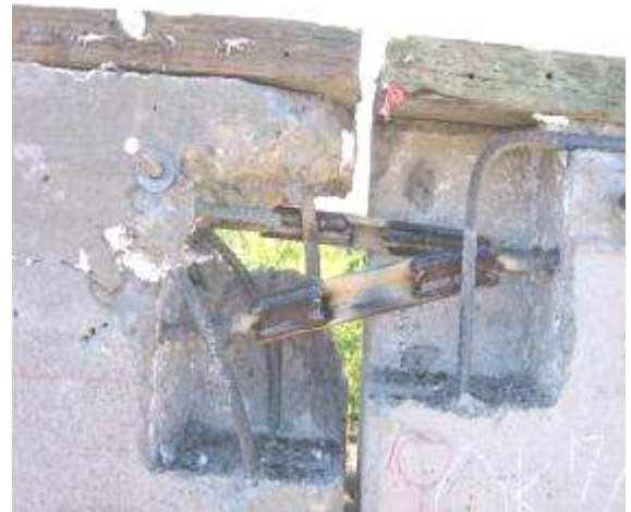
Figure 2-17: Poor Layout for Chord Steel
