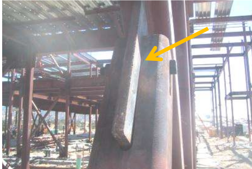
Figure 2-60: Erection Bolt Closing HSS Gap
