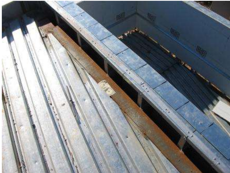
Figure 2-51: Skewed Deck Edge Modifies Perimeter Welding Requirements
